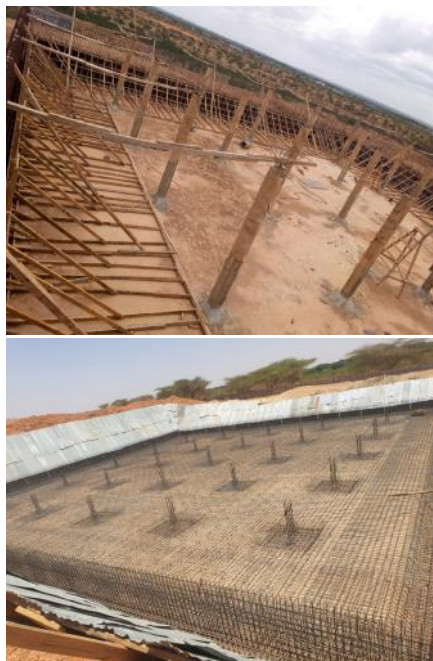
Water treatment tanks in Shashafey 5 million litres capacity
